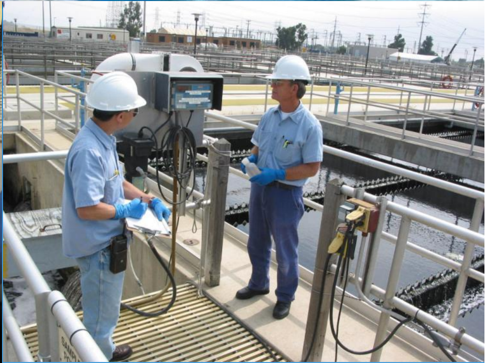
Treatment plant designed for maximum reclamation
